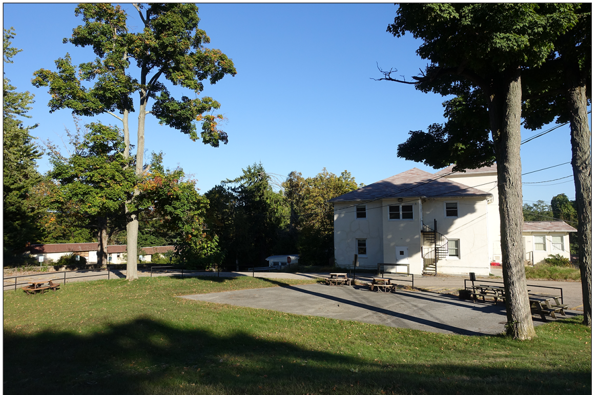
View on South Building and Recreation Building 4
