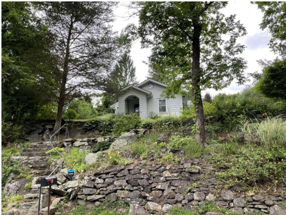
Front view. Proposed addition would go on right side of photograph.
