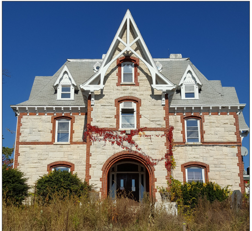
Facing northeast from south of the Main Building. Building is located at top of hill
