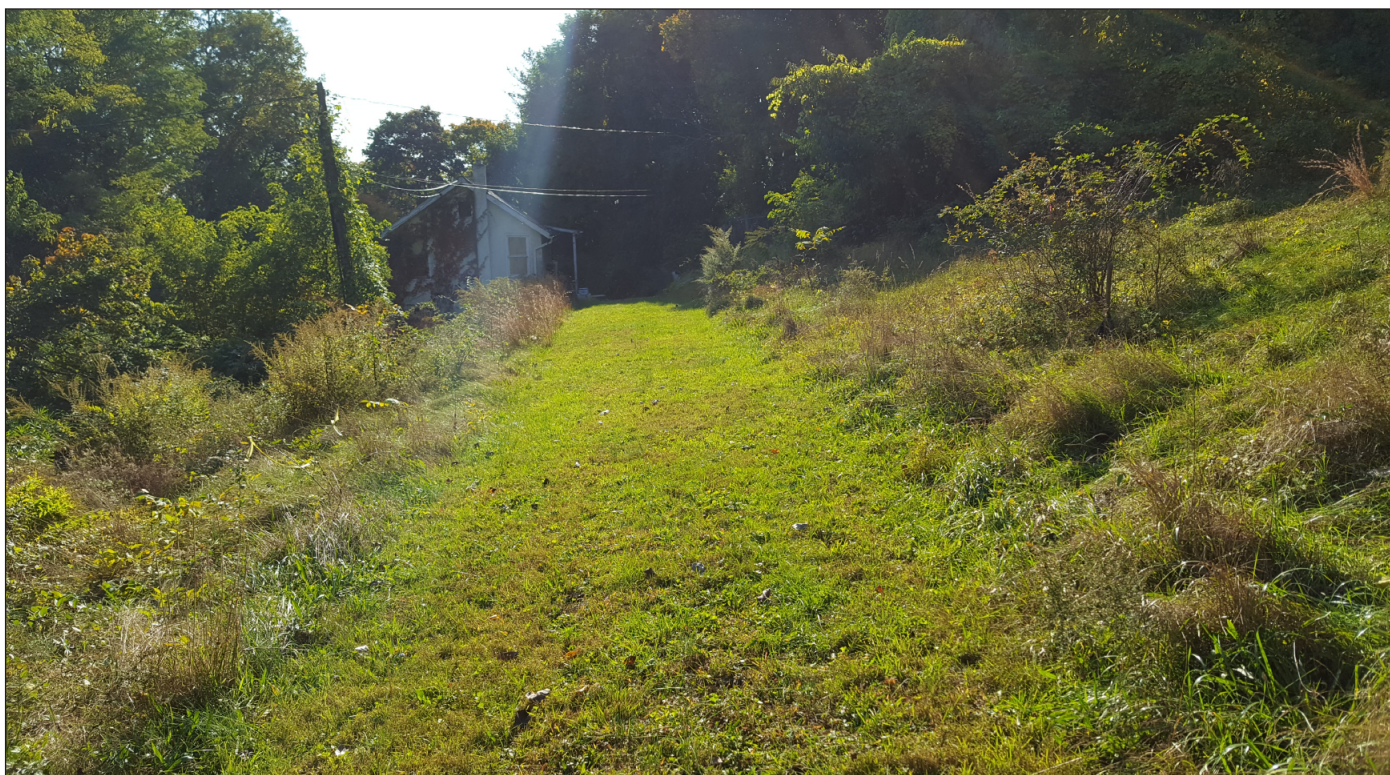
Facing southwest along southeastern edge of Project Area showing level area at base of hill and Maintenance Building. Note wetland area on the left 20
