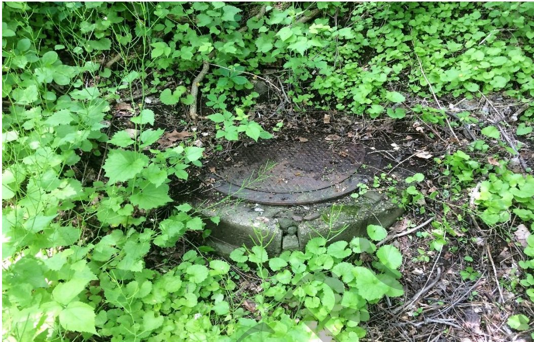
Photo 9: Subsurface infrastructure was noted in the northeastern portion of the site. View to the northeast.
