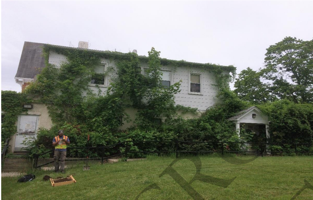
Photo 3: Additions have been constructed on the rear of the Main Building. The level lawn to the north of the house is considered archaeologically sensitive. View to the south of TR 1.
