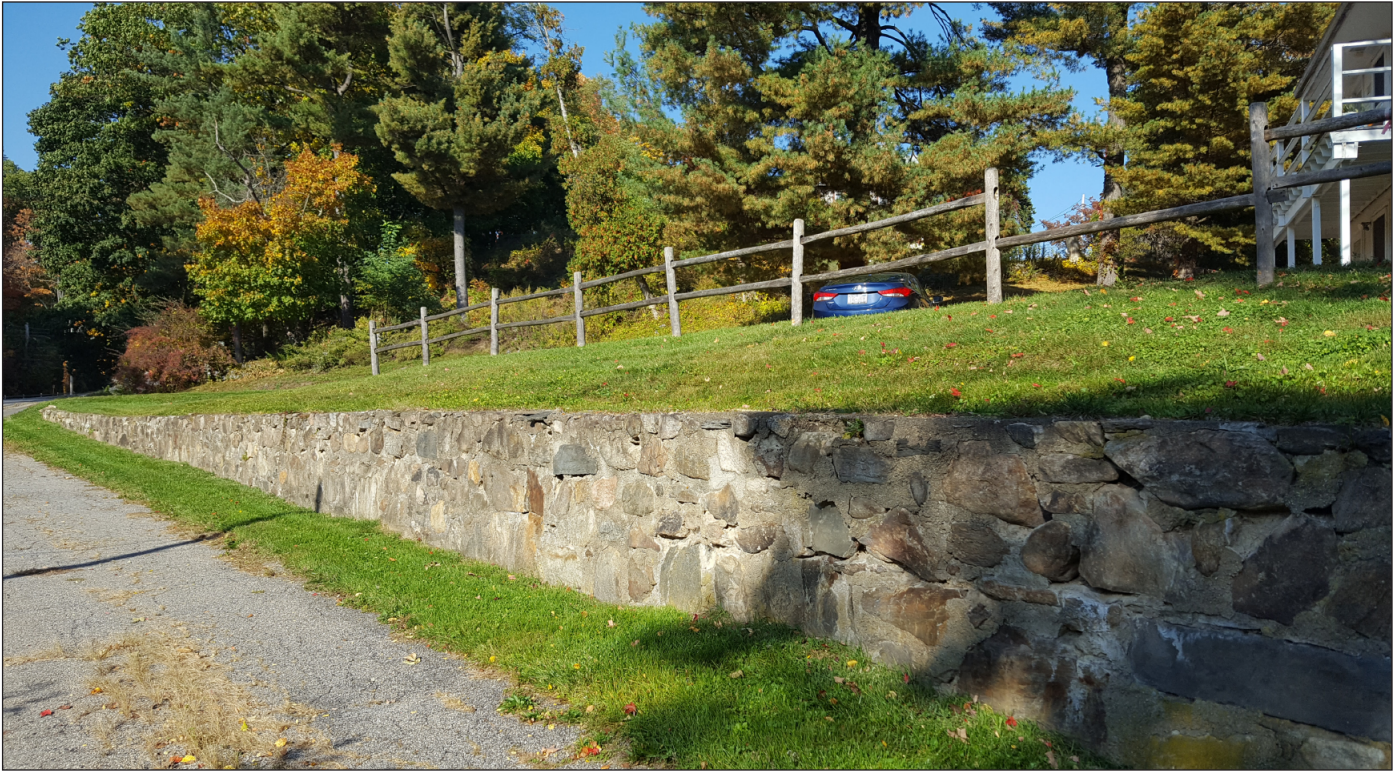
Facing north along driveway in western corner of project Area showing stone retaining wall and rising topography 11
