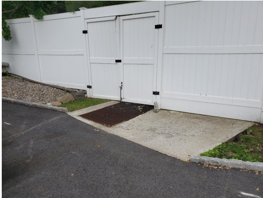
Figure 1: Catch Basin on the Property
