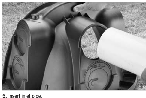
5. Insert inlet pipe.
