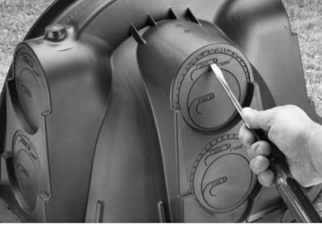
1. Start tear-out seal.
